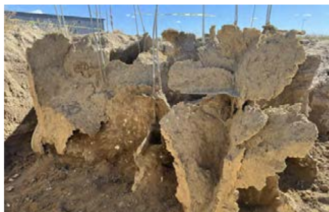
Figure 9: Posttreatment excavation-clay site
