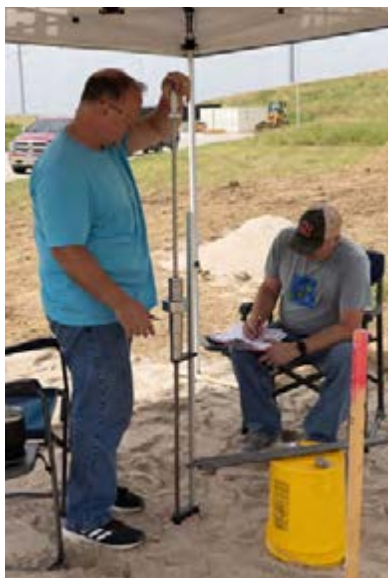
Figure 1: DCP testing at the sand site
